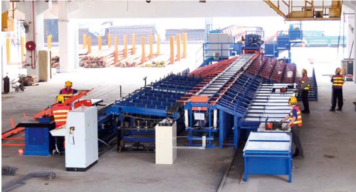
Rebar Value-Added Centre in Tai Po, Hong Kong
