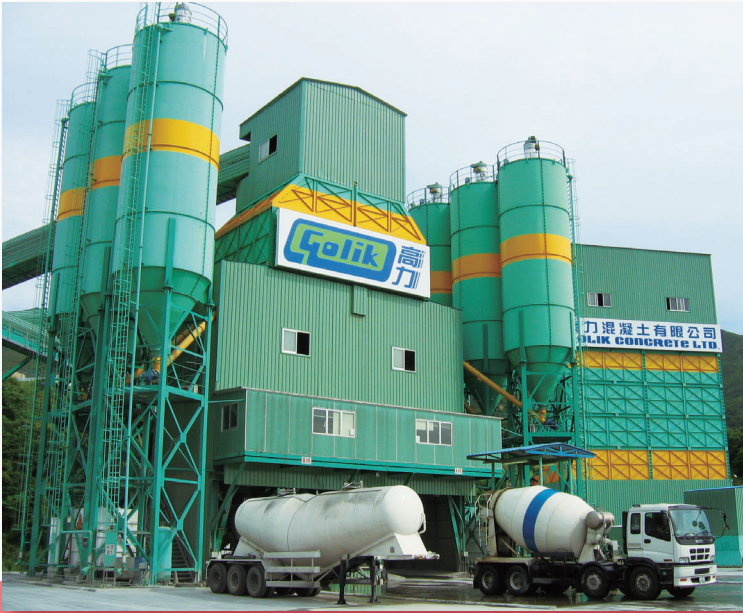
Ready Mixed Concrete Plant in Siu Ho Wan, Lantau Island, Hong Kong
