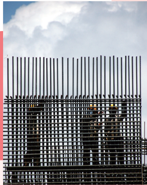
Steel Reinforcement Bars – Application on construction site
