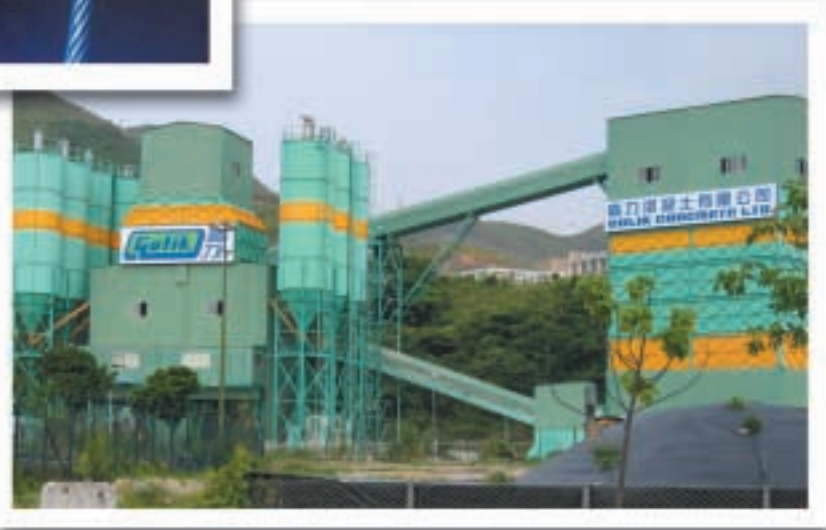
Ready Mixed Concrete Plant in Siu Ho Wan, Lantau Island, Hong Kong
